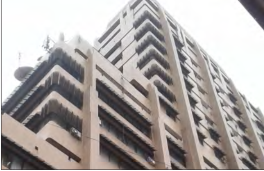
Figure 6: Gécamines Tower, sunshades. © Author, 2015
