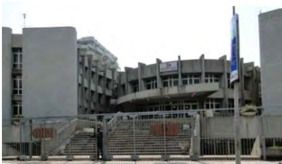
Figure 7: OGEDEP building by Magema. © Author, 2015
