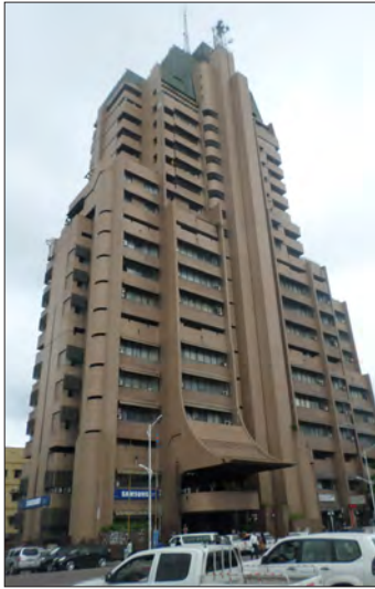
Figure 4: Gécamines Tower. © Author, 2015
