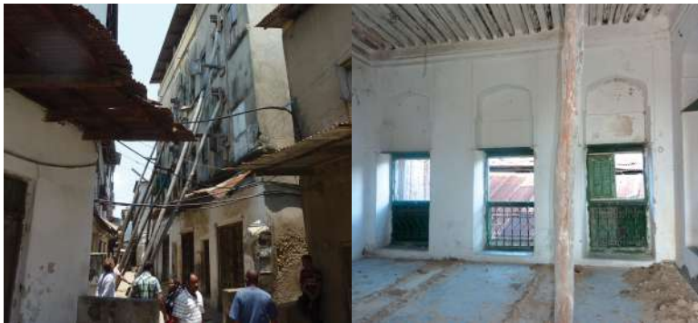
Fig.8 & 9: Exterior and interior of the building
